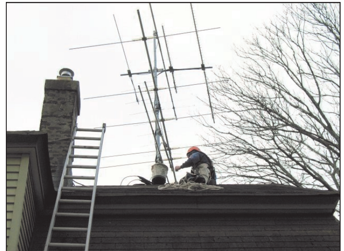
Finishing off the 1296 hardline installation
